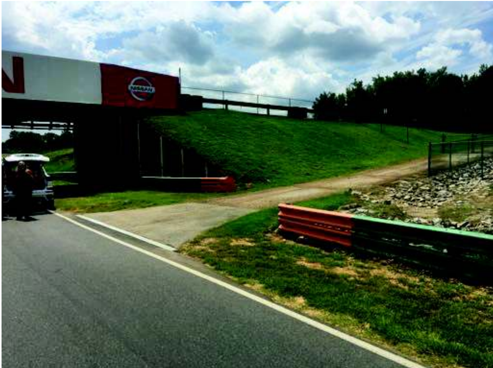
Nissan Bridge, Drivers Right
